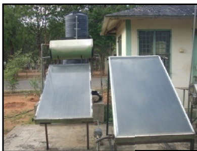
Solar Water Heater-Flat Plate Collector
